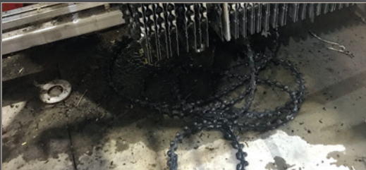
Loose gaskets during field cleaning services
